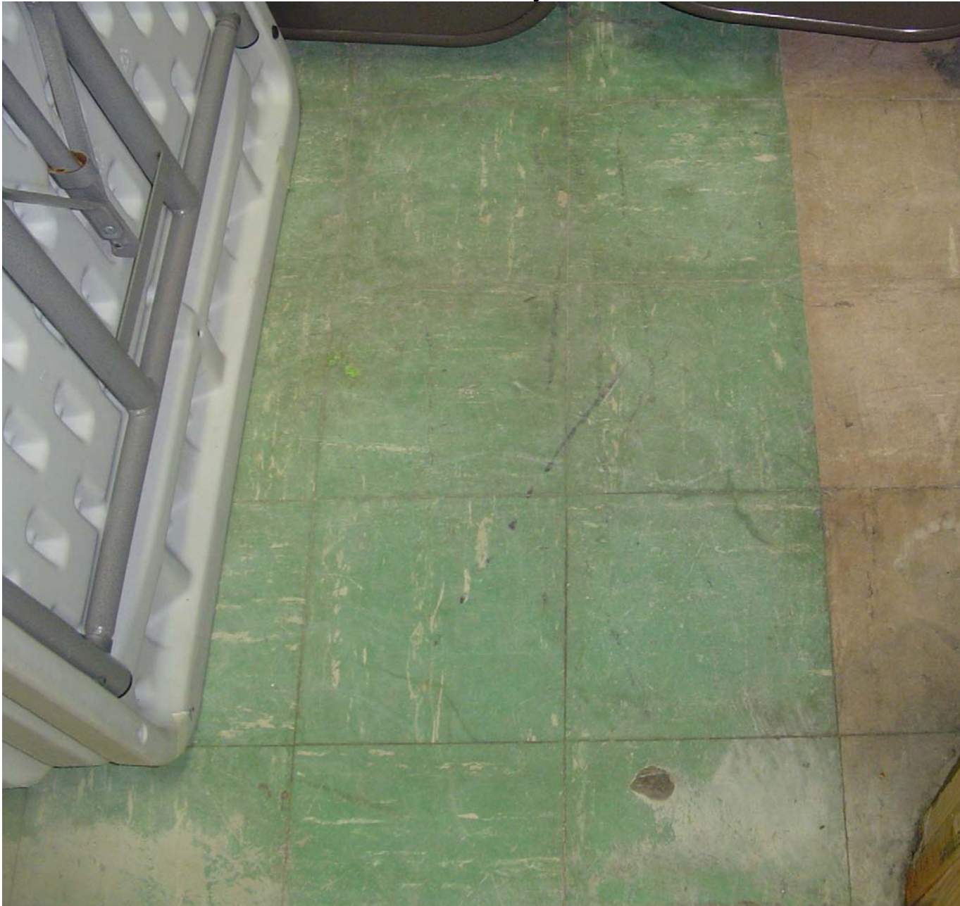
9"X9" green floor tile and mastic (covered by floor tile) throughout the Gymnasium Building
