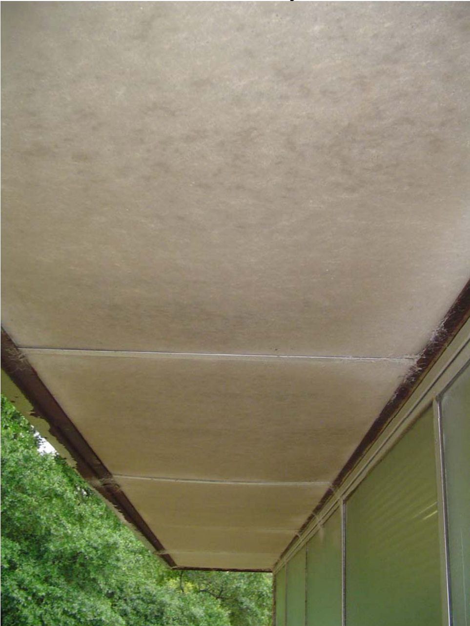
Exterior gray soffit panels throughout Buildings A – E, H, I, and the Main Office Building
