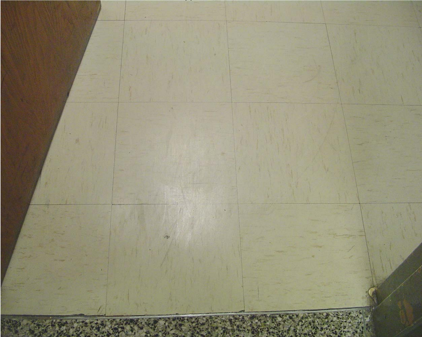
12"X12" off-white floor tile in Classrooms 115 – 119 and 210 – 218
