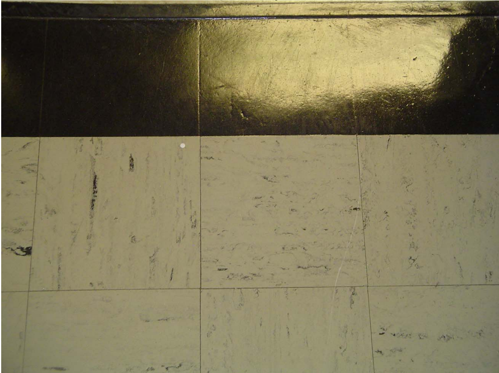
9"x9" off-white floor tile, 9"x9" black border floor tile, and mastic in the Cafeteria, Classrooms 5, 6, and 29, Teachers Lounge, Safe, Lobby, & throughout hallways
