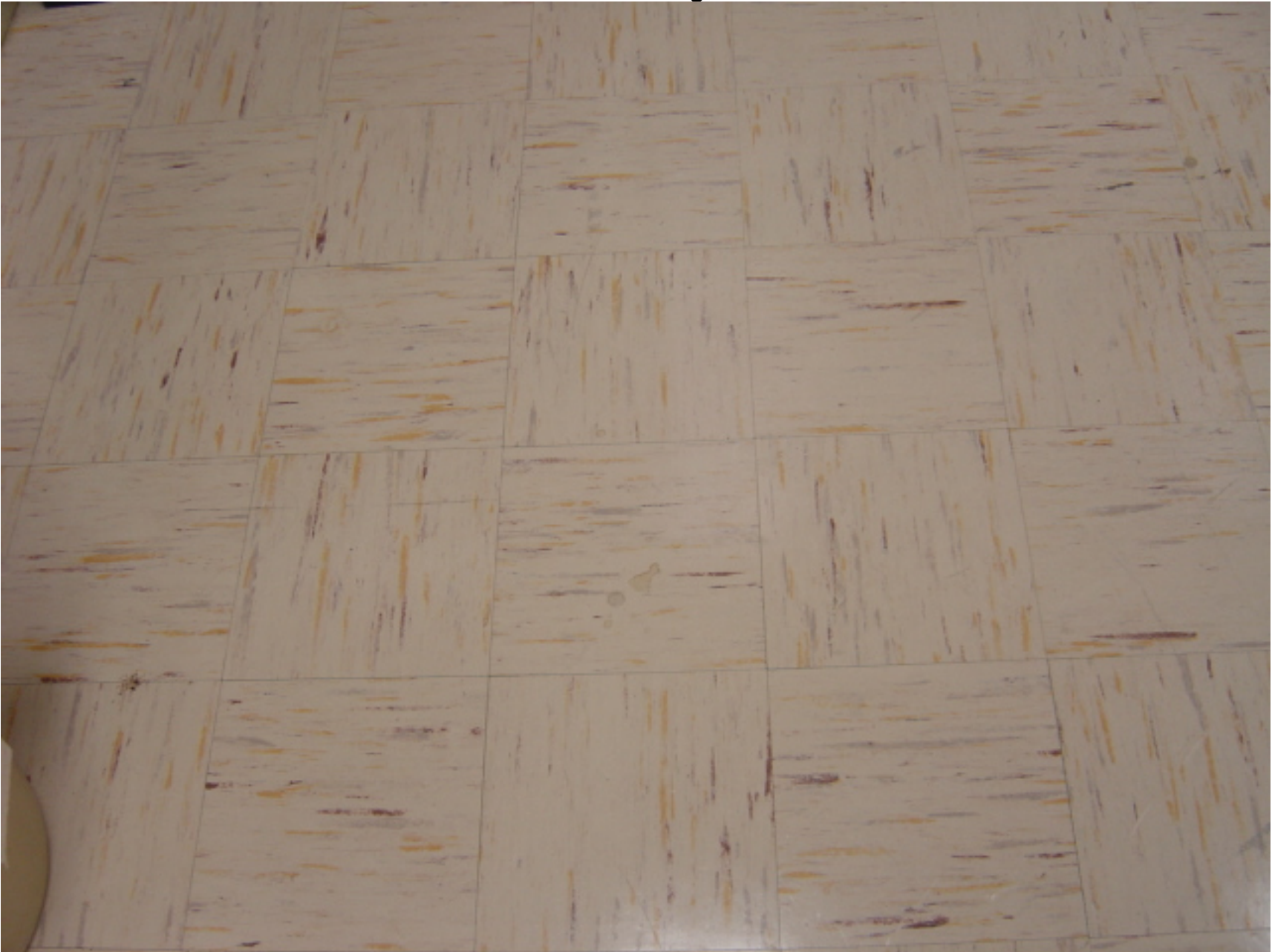
9"X9" tan floor tile and black mastic throughout the Main Facility
