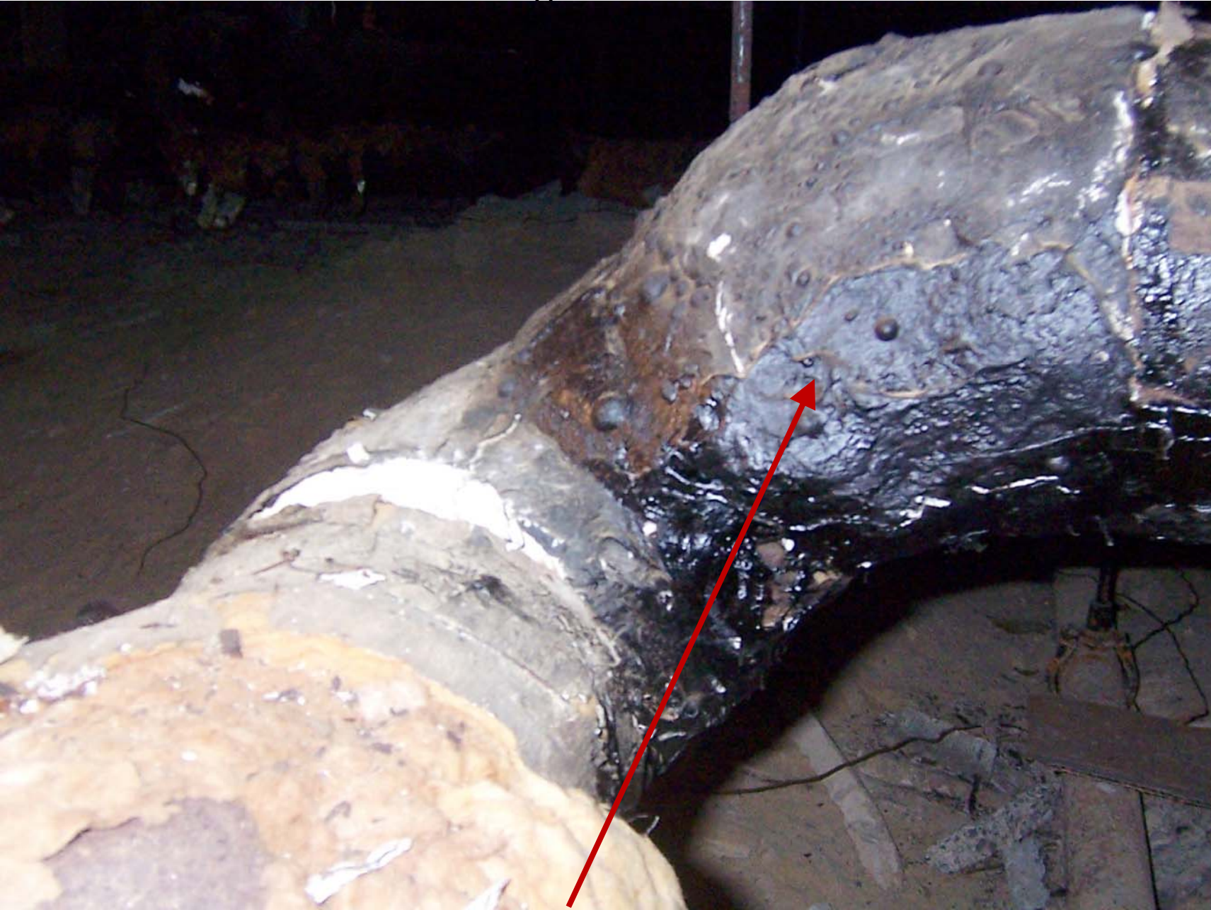
Hard pipe insulation elbows and tar throughout the Main Facility crawlspace
