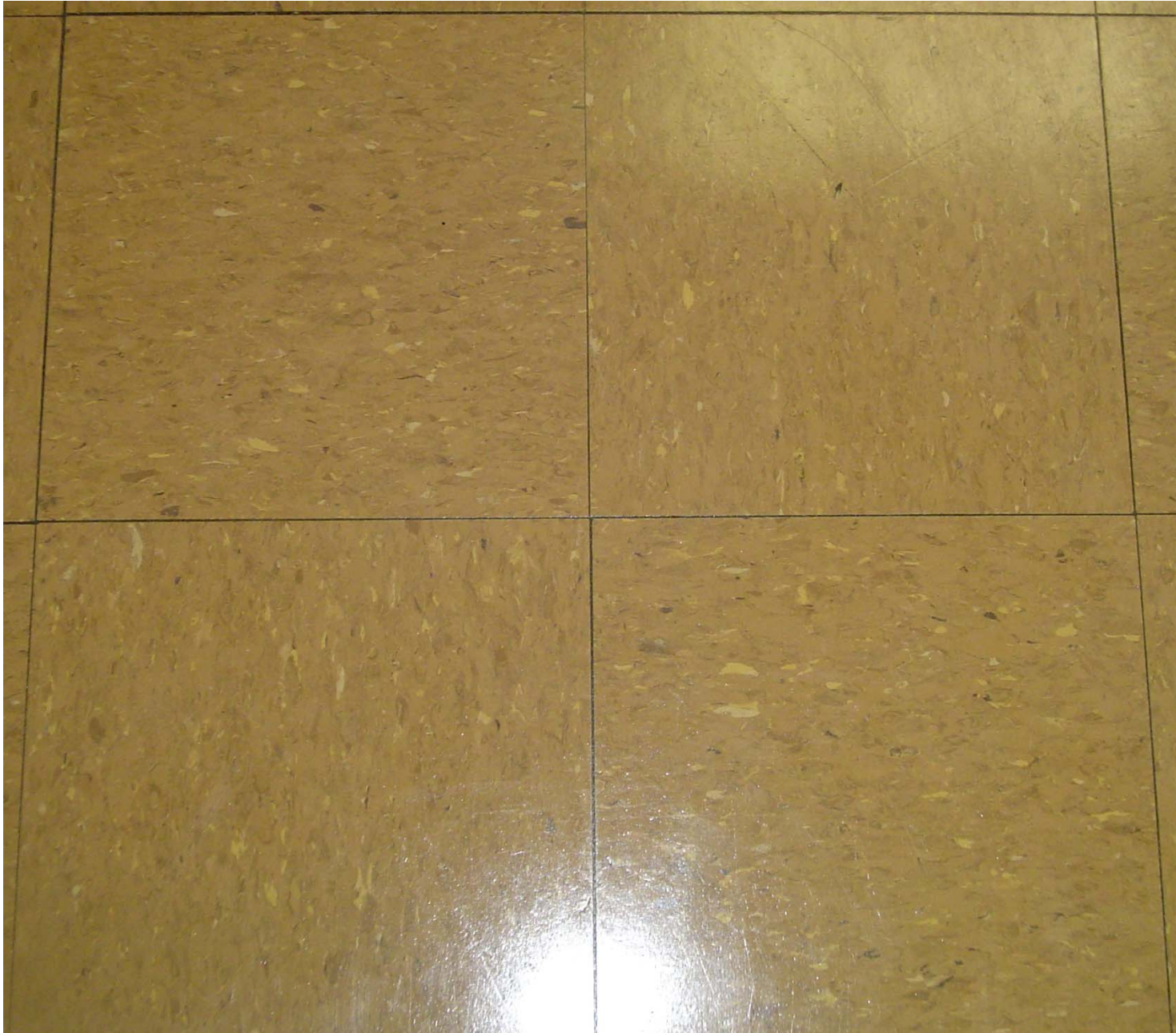
12"X12" dark tan floor tile and black mastic throughout the Main Facility
