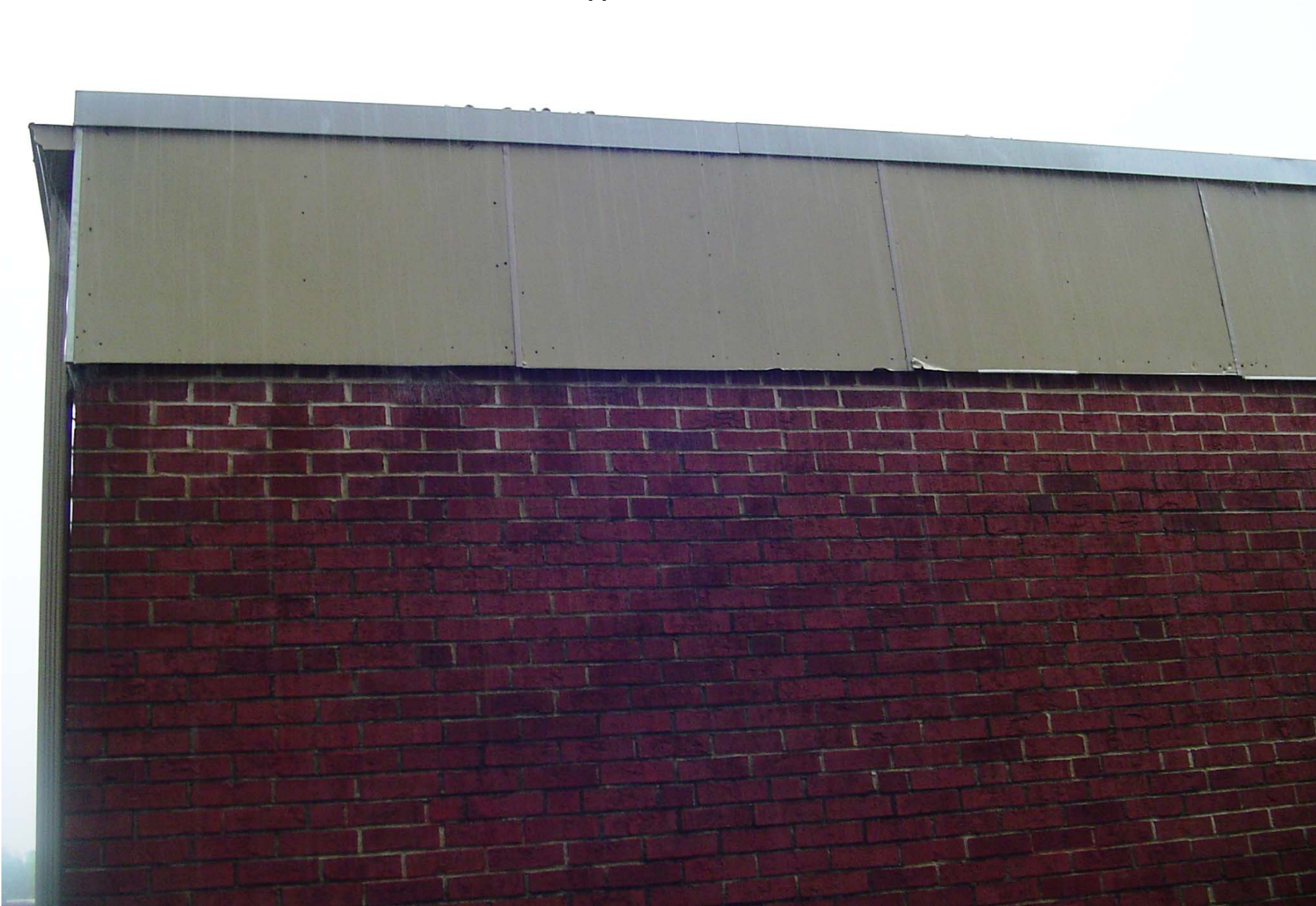
Exterior light tan transite panels below the roofline around the Annex Building II – Testing and Servers (1970 Building)
