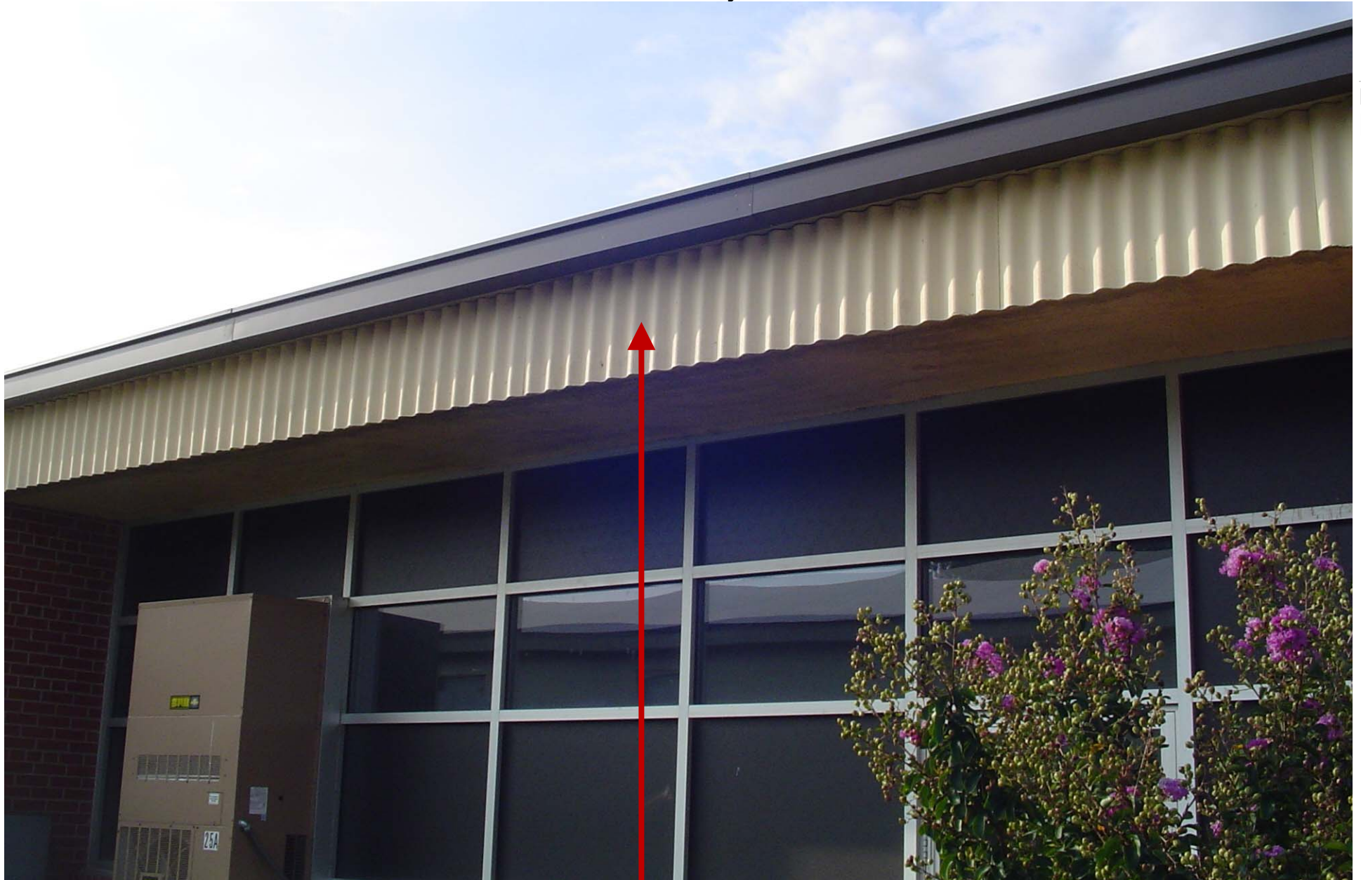
Exterior white decorative fascia border below the roof line around the 300 Wing
