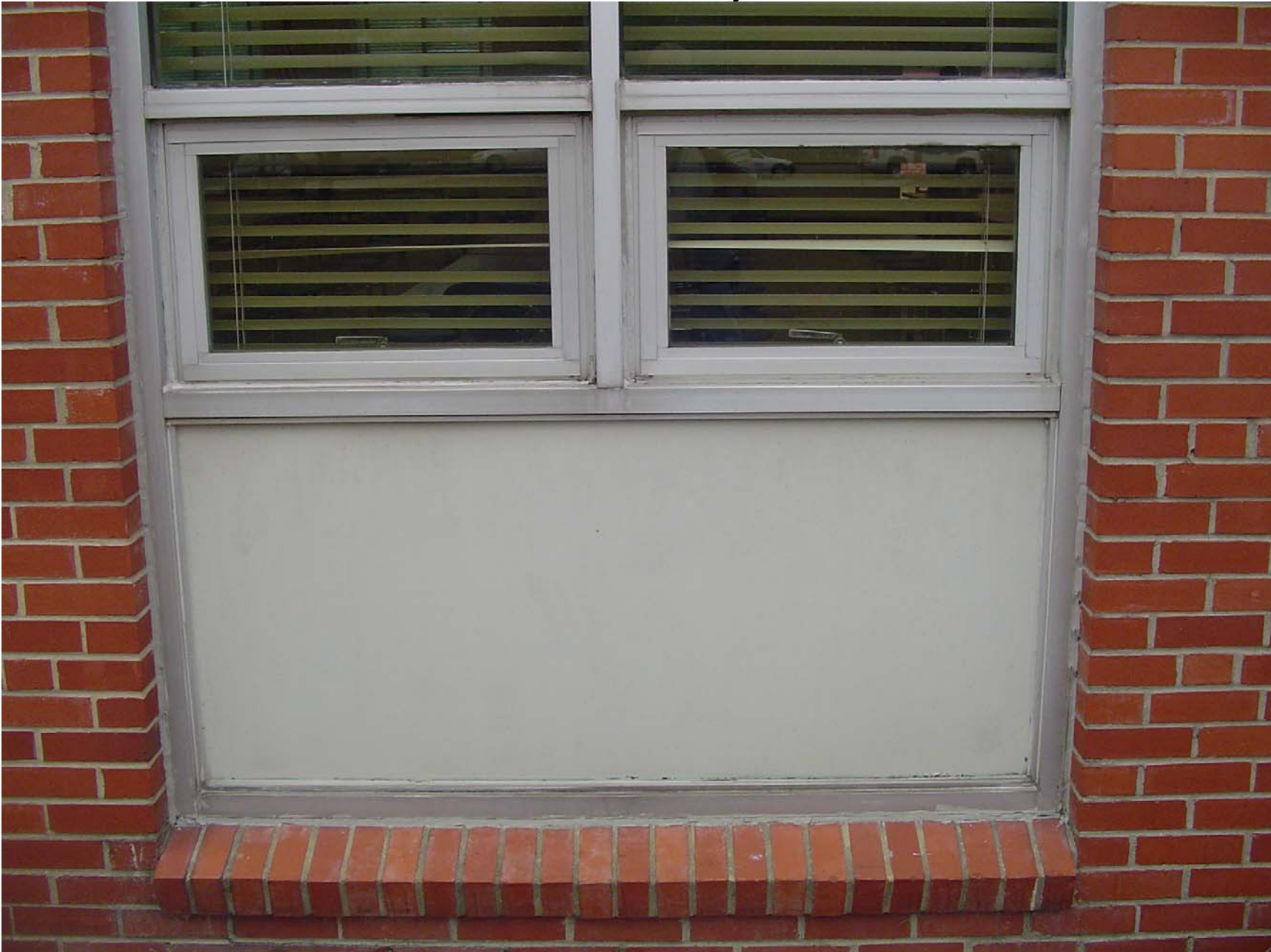
Transite Panels below the windows in the Cafeteria
