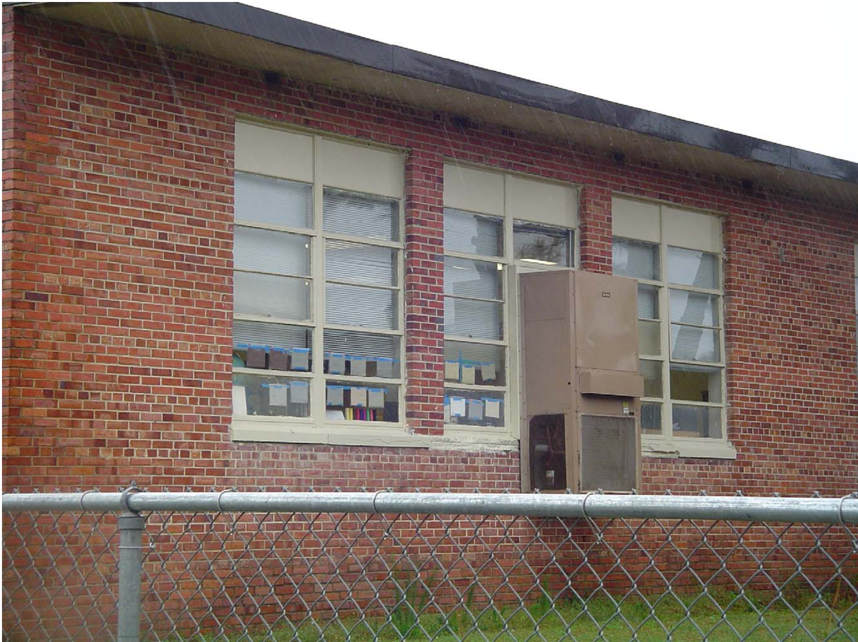
Exterior window glazing in Classrooms 404 and 506 – 508
