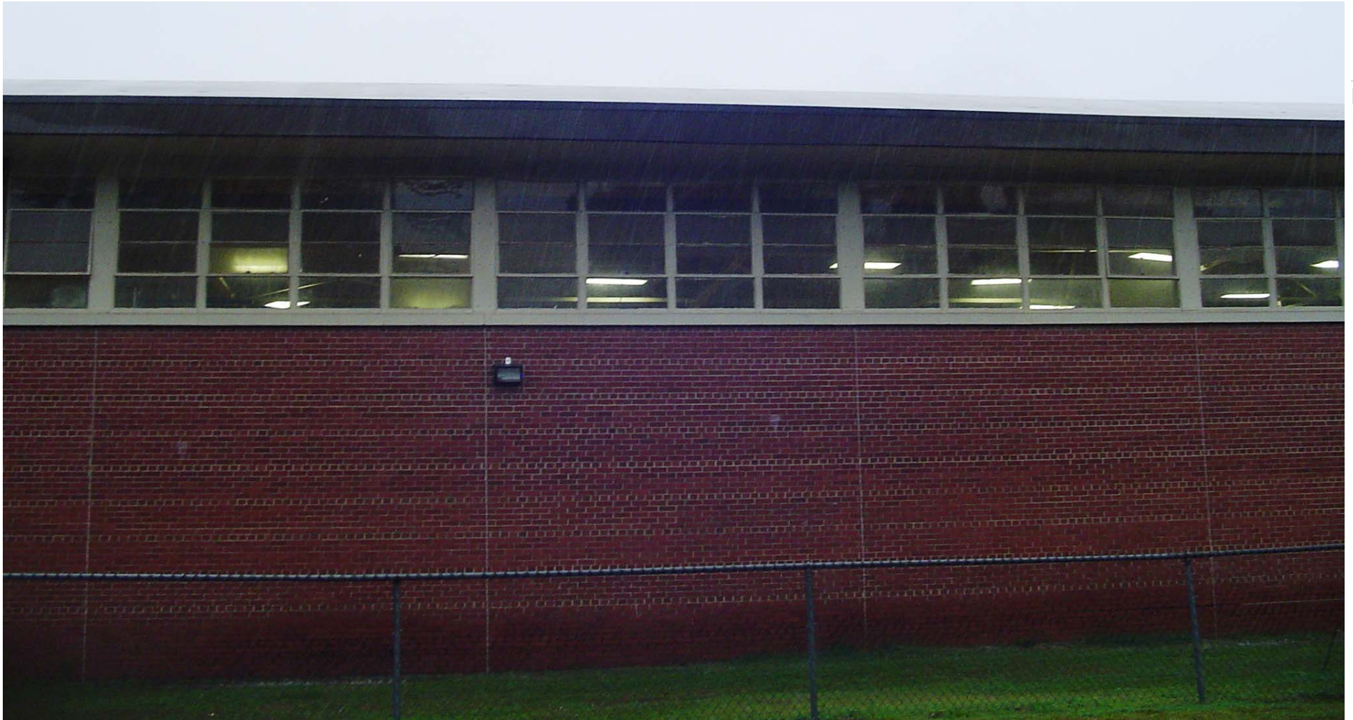
Exterior window glazing in the Gymnasium
