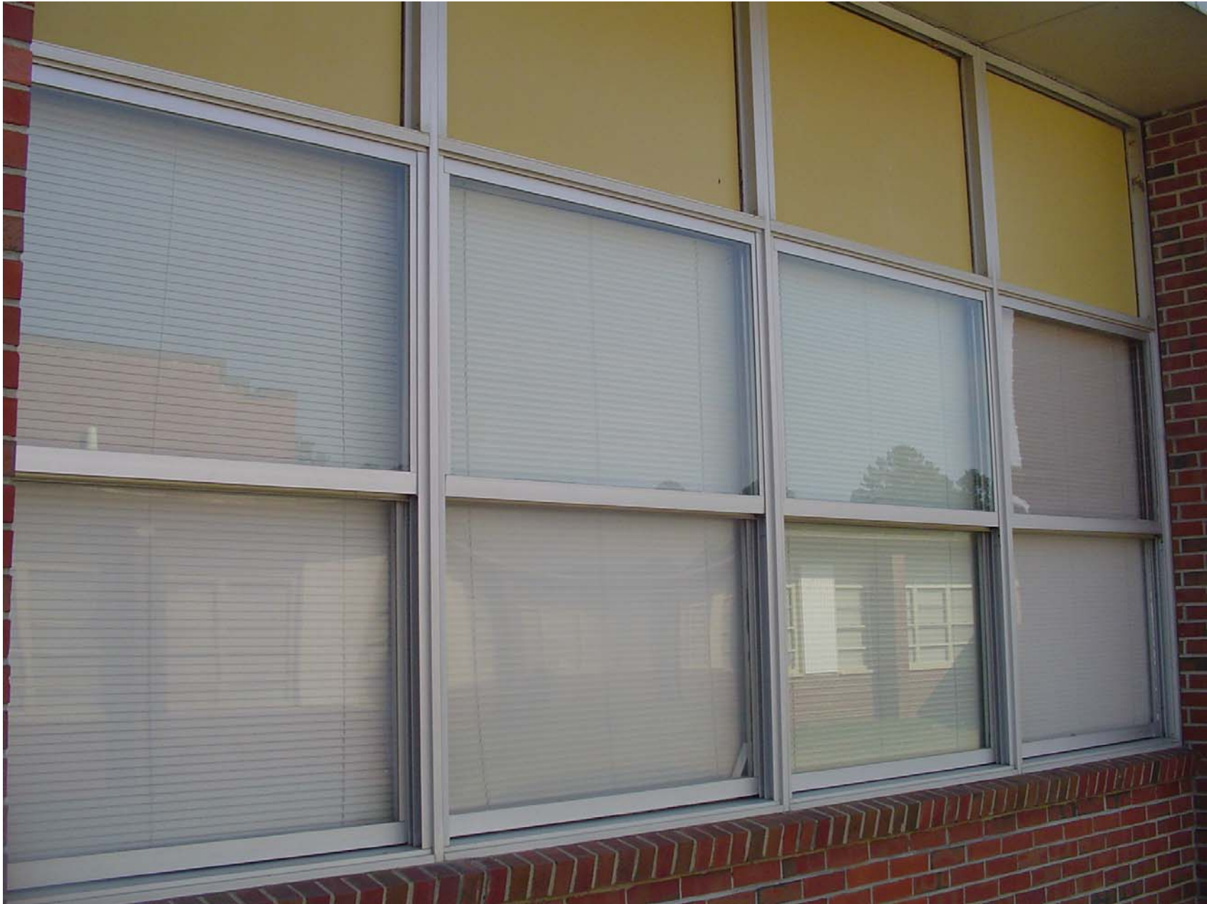
Exterior window glazing and transite panels throughout the old section of the 200 Wing
