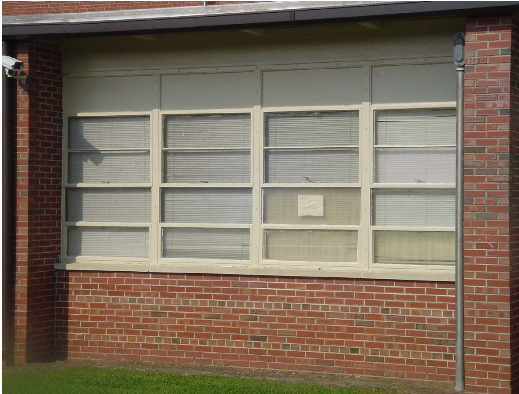
Exterior window glazing throughout the 120 Wing
