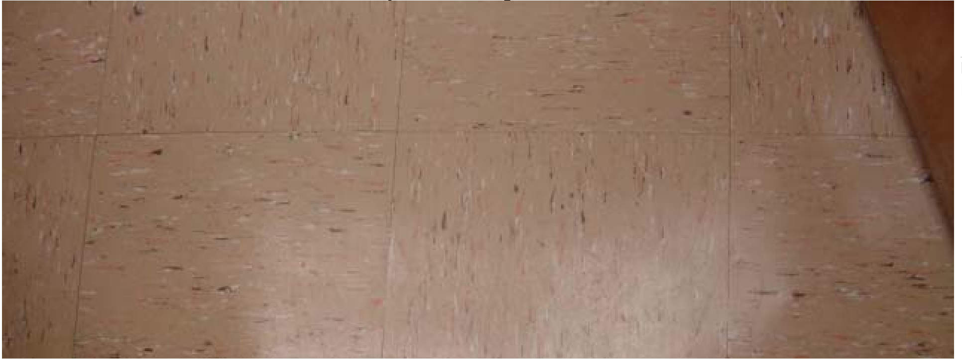
12"X12" beige floor tile and black mastic throughout the Main Facility
