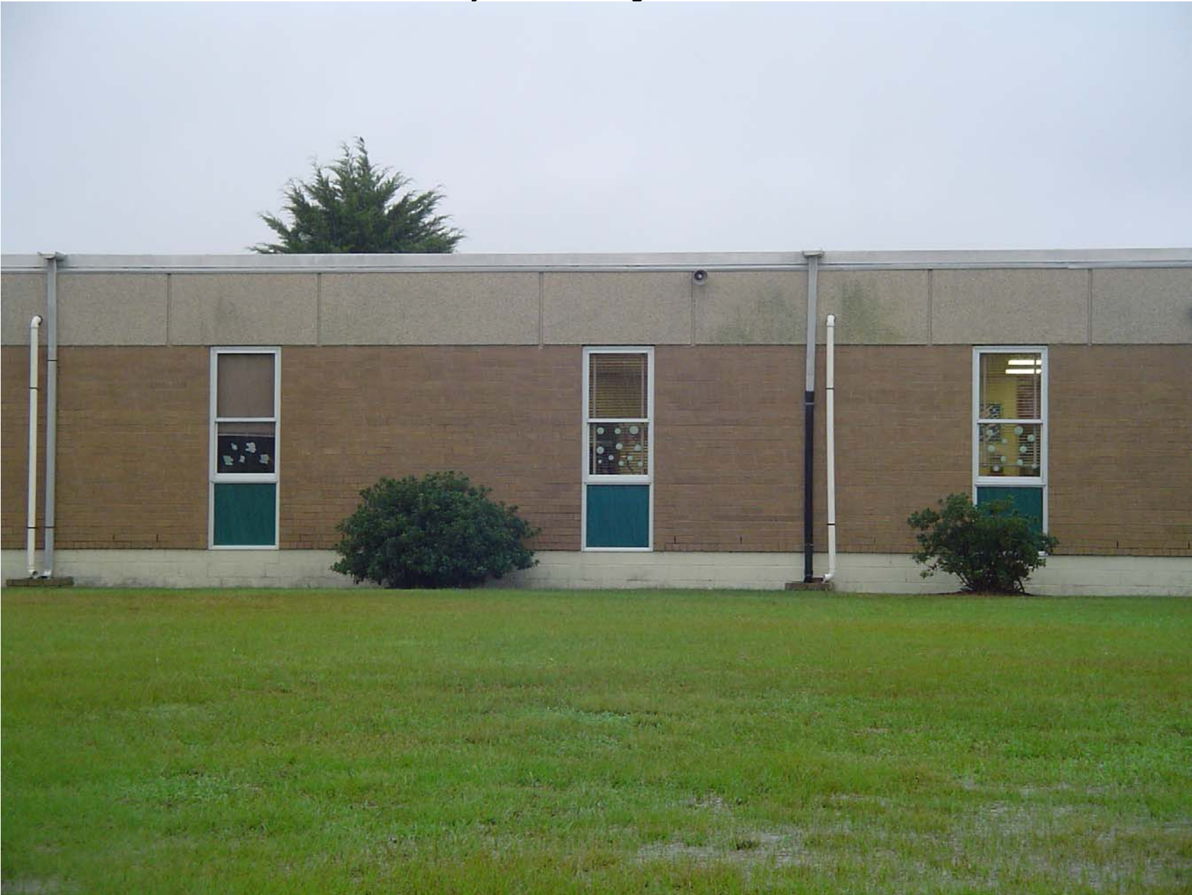
Window glazing and transite panels throughout the Main Facility
