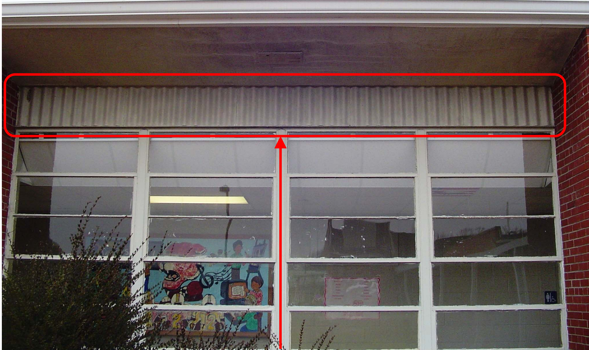
Exterior decorative trim below the roofline of the 600 Wing
