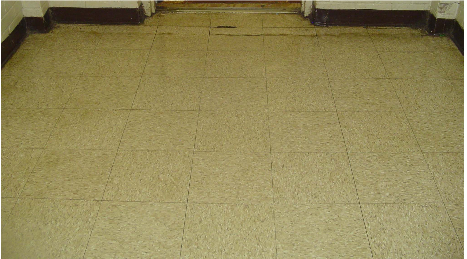
12"X12" brown floor tile and black mastic in the hallway between the locker rooms
