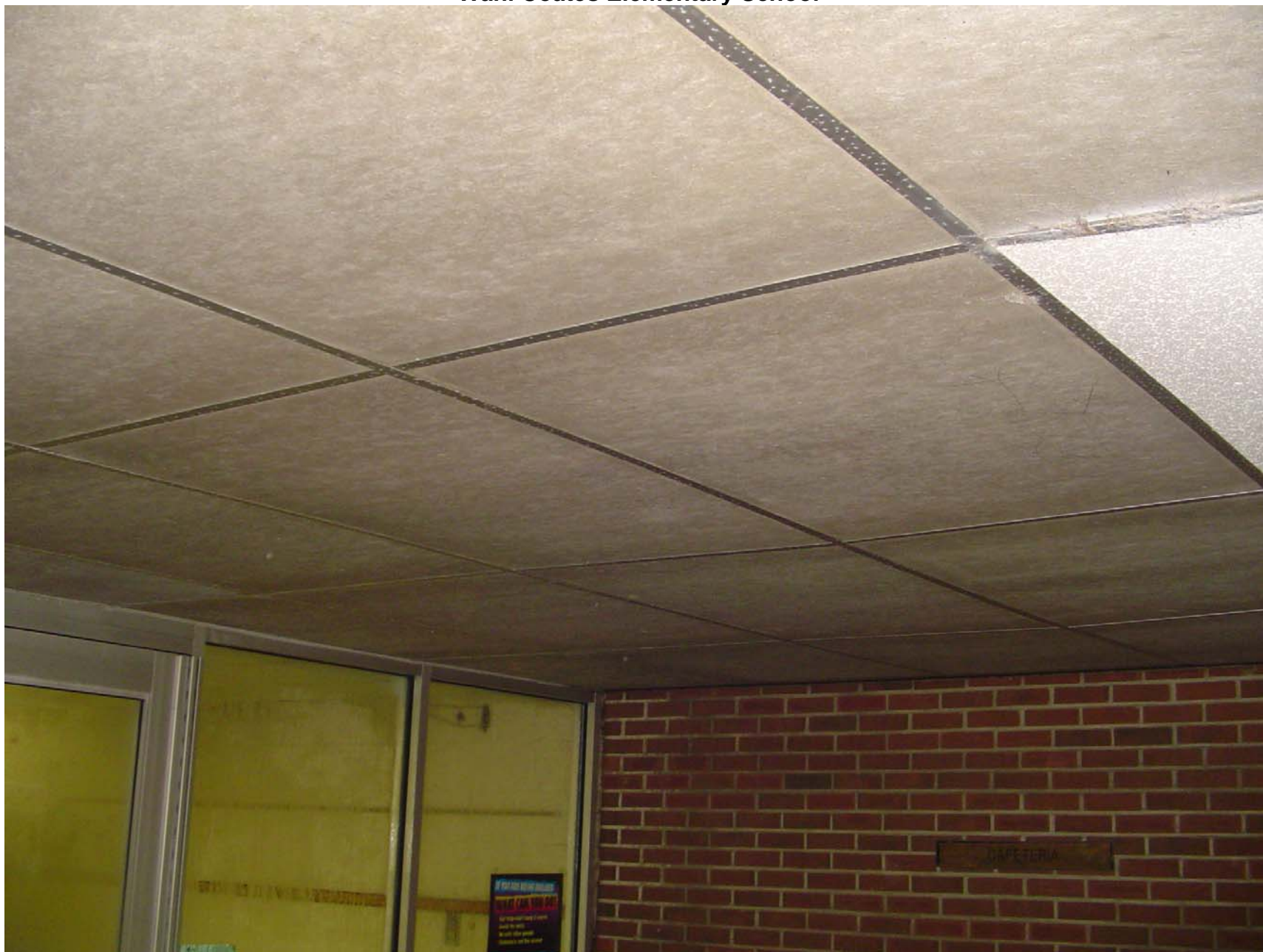
Exterior 32”X48” exterior ceiling tiles under the canopies throughout Buildings E, H, I, and the Cafeteria
