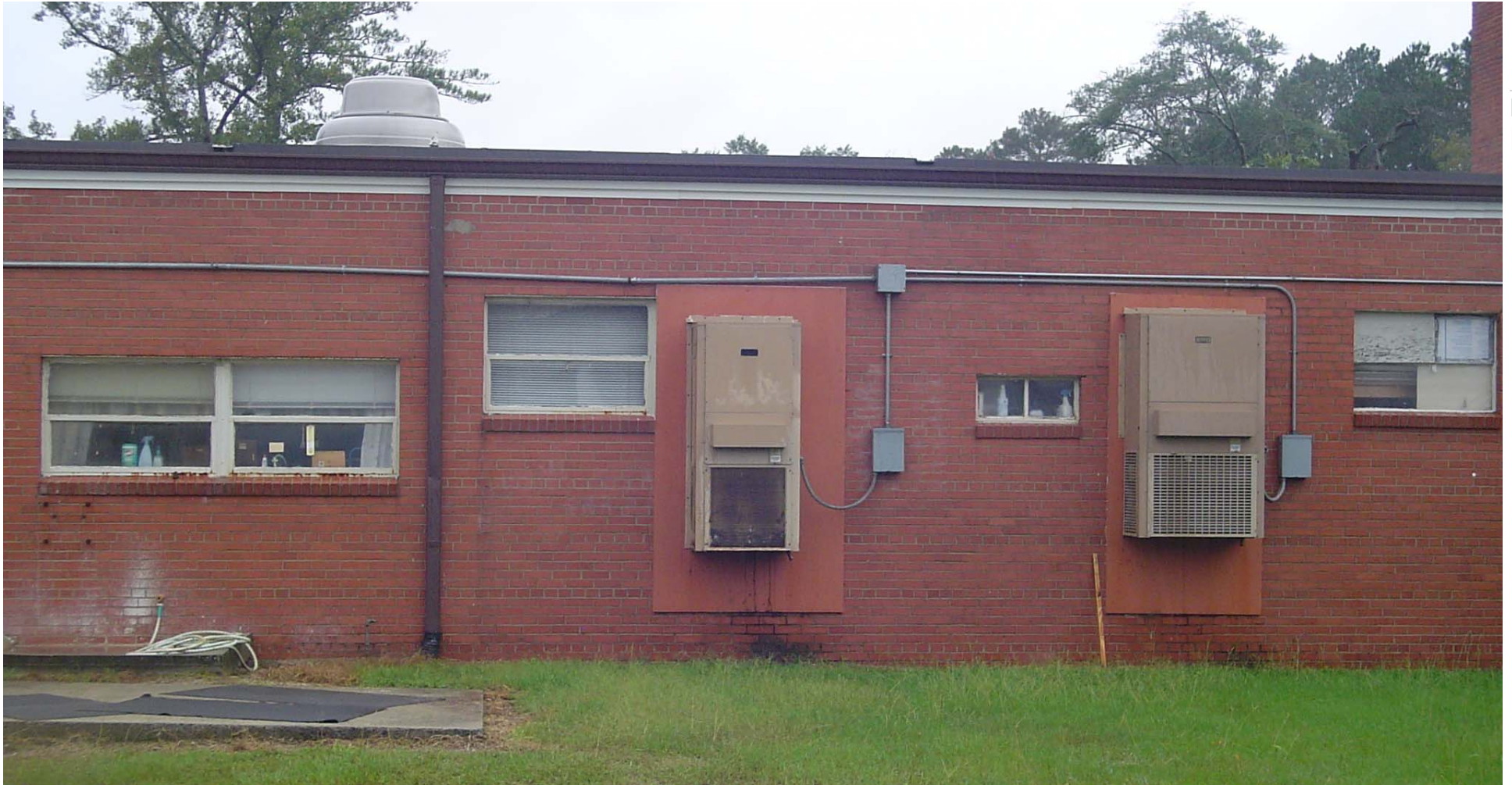
Window glazing in Classrooms 103, 105, and 107
