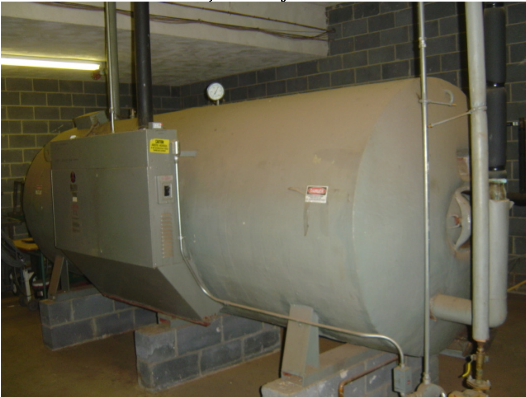
Insulation located on hot water tank in the Main Mechanical Room
