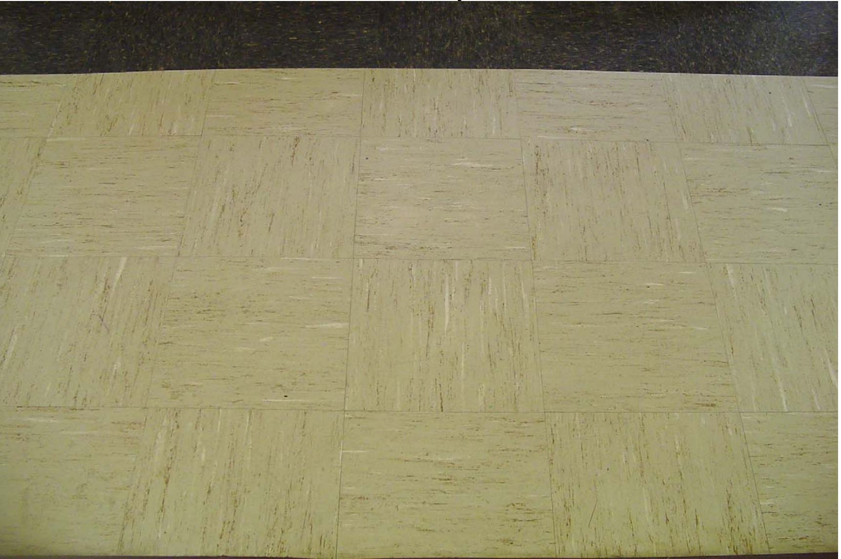
12"X12" light tan floor tile (partially covered by carpet) in Classrooms 103 and 105
