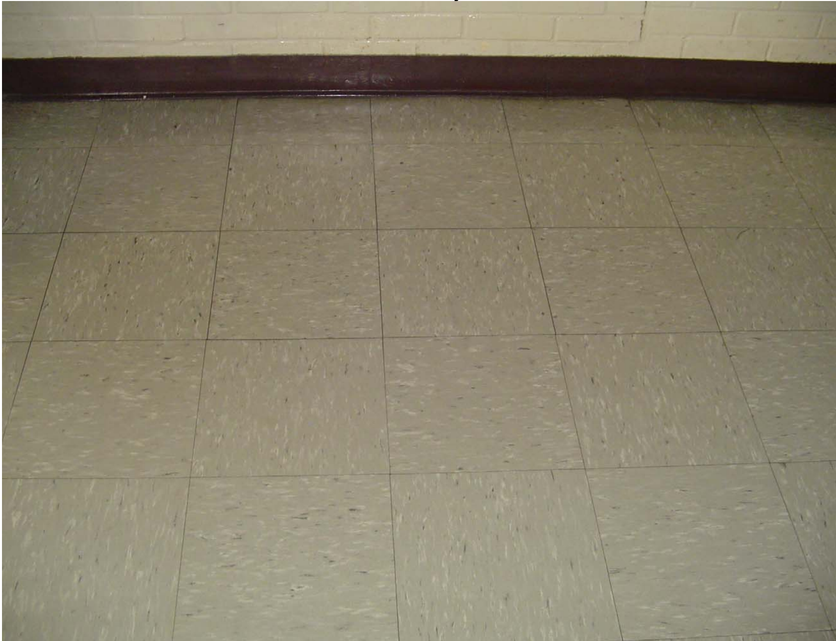
12"X12" gray floor tile and black mastic in the Cafeteria and adjoining hallway
