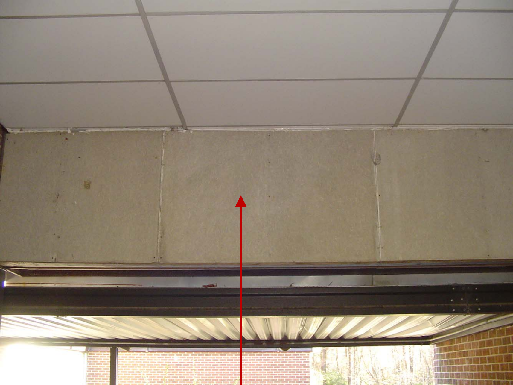
Exterior gray fascia panels below the roofline around Buildings E and H, Cafeteria, and the Gymnasium
