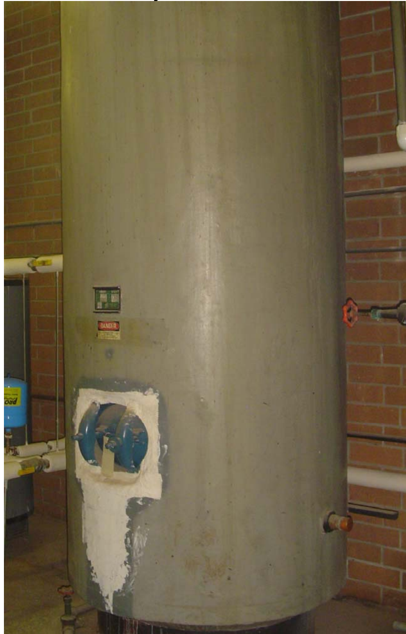
Insulation located on the hot water storage tank in the Boiler Room
