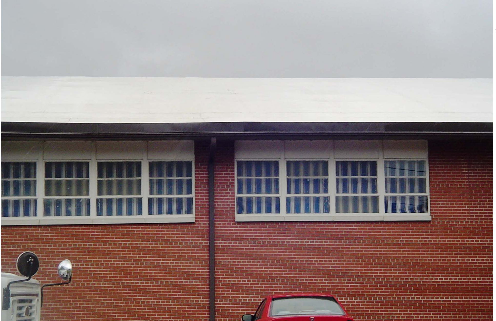
Exterior window glazing throughout the Gymnasium Building
