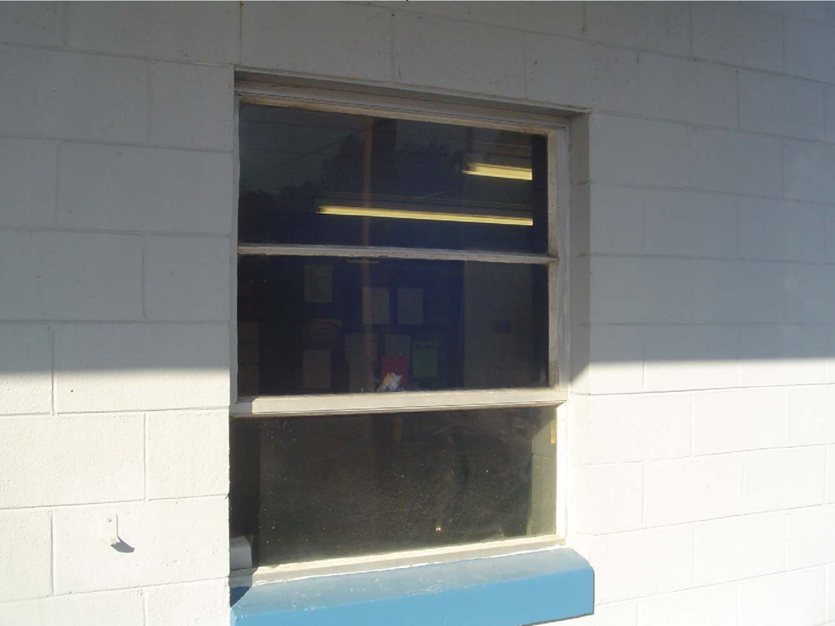
Exterior window glazing throughout the Main Facility
