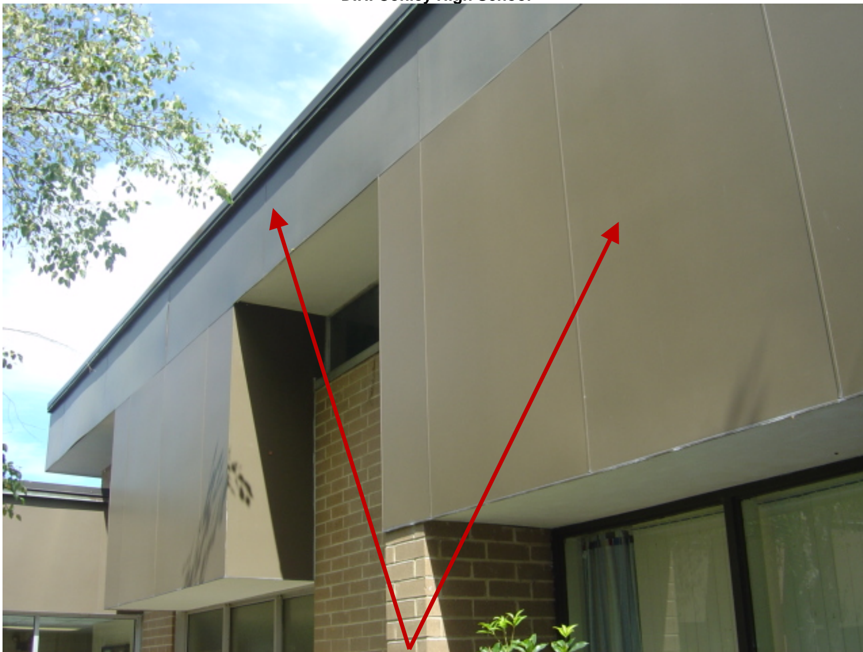
Exterior dark brown transite panels of various sizes below the roofline at various locations around the Main Facility
