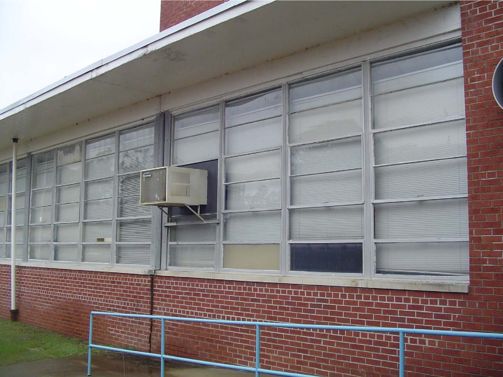
Exterior window glazing throughout the Main Facility
