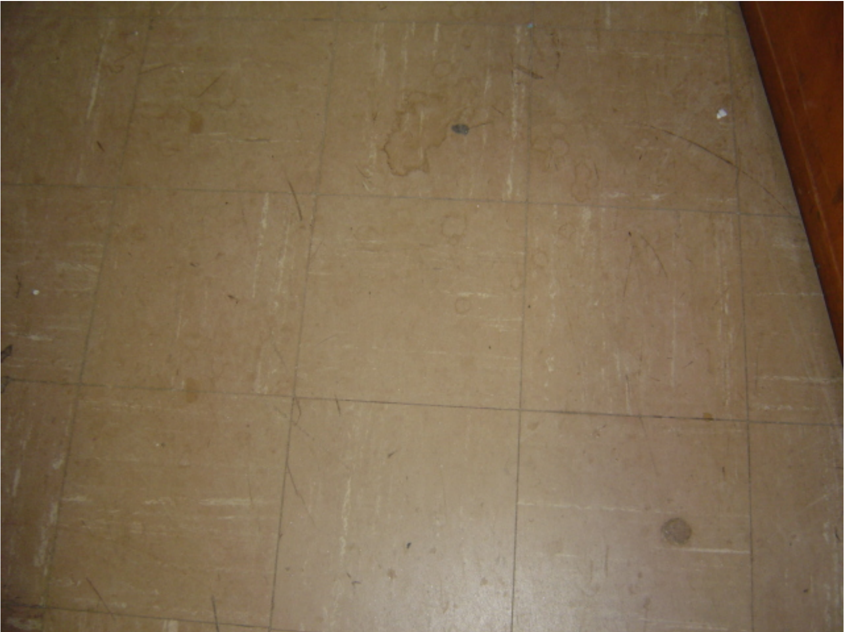
9"X9" light brown floor tile and black mastic in the Athletic Storage Room in the Gymnasium
