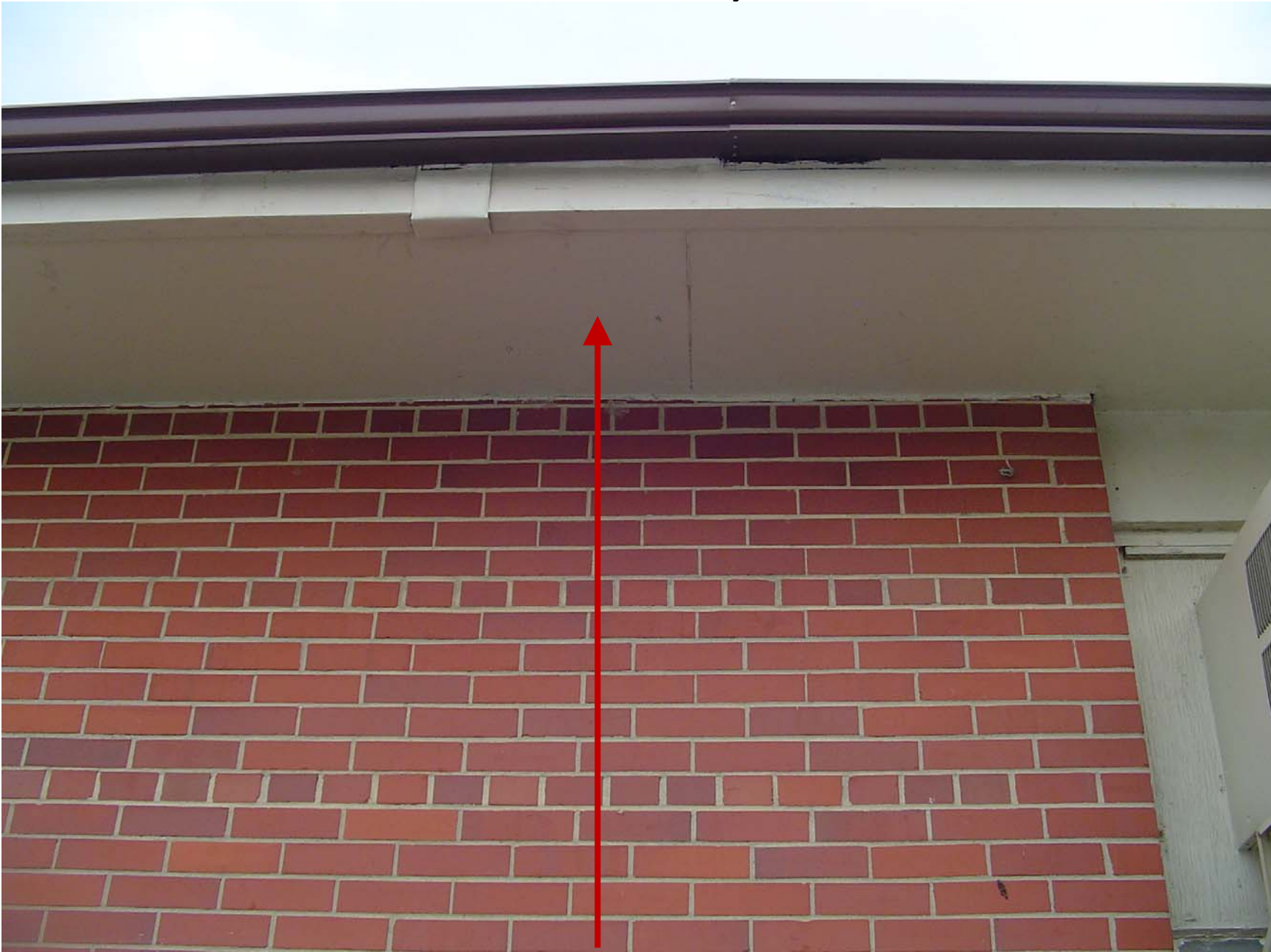
Exterior soffit panels High section of the Gymnasium and the low, back side of the Gymnasium
